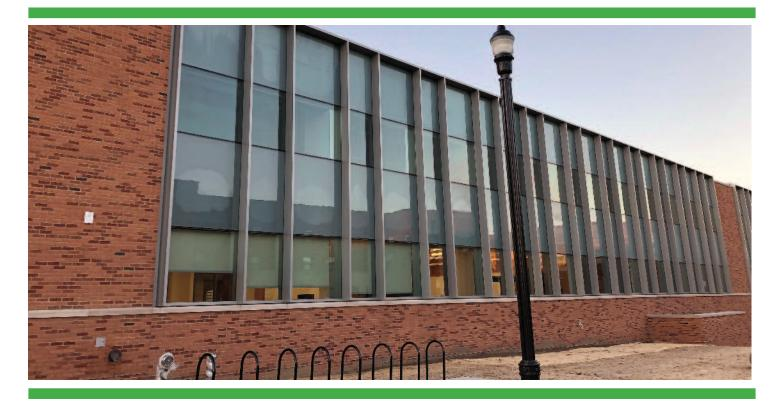
Exterior building materials - brick and aluminum/glass curtain wall - were selected to harmonize with the other buildings of the science complex, and were detailed for durability and energy efficiency.
